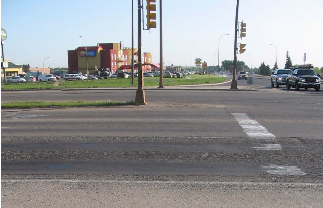
Photo 1: Rutting at the stop bar on Hwy 1 at Dunmore Road Intersection. Note that the surface had been milled to address rut depth. A thin layer of new ACP was required every 2 nd year to provide a smooth driving surface.
