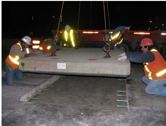
Figure 10 Highway 427 Full Depth Repair-Precast Concrete
