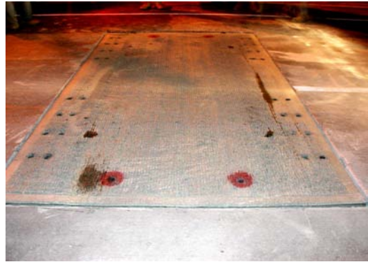
Figure 10 (cont'd): Highway 427 Full Depth Repair-Precast Concrete
