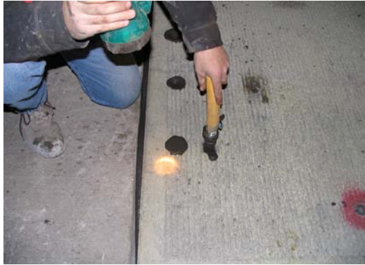
Figure 10 (cont'd): Highway 427 Full Depth Repair-Precast Concrete
