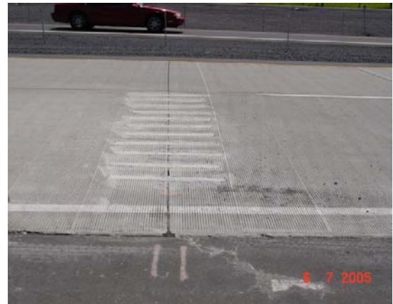
Figure 9 Highway 417 Westbound Dowel-Bar retrofit
