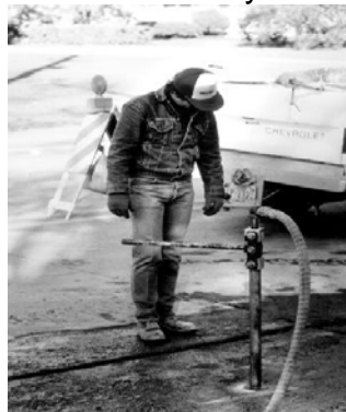
Figure 6 Slab Stabilization/Jacking [ACPA-TB020P]
