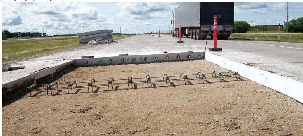
Figure 12: Highway 75 Full Depth Repair Winnipeg, Manitoba [IGGA March 2010]
