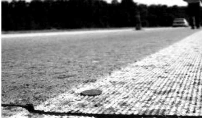
Figure 3: Diamond Ground Surface [ACPA-TB020P]
