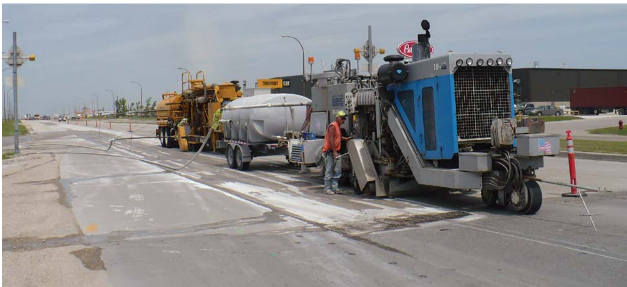
Figure 11: Diamond Grinding Test and Trial Project in Winnipeg, Manitoba [IGGA January 2010]
