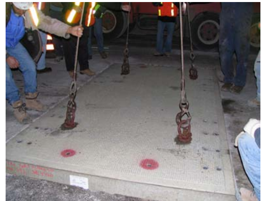
Figure 10 Highway 427 Full Depth Repair-Precast Concrete
