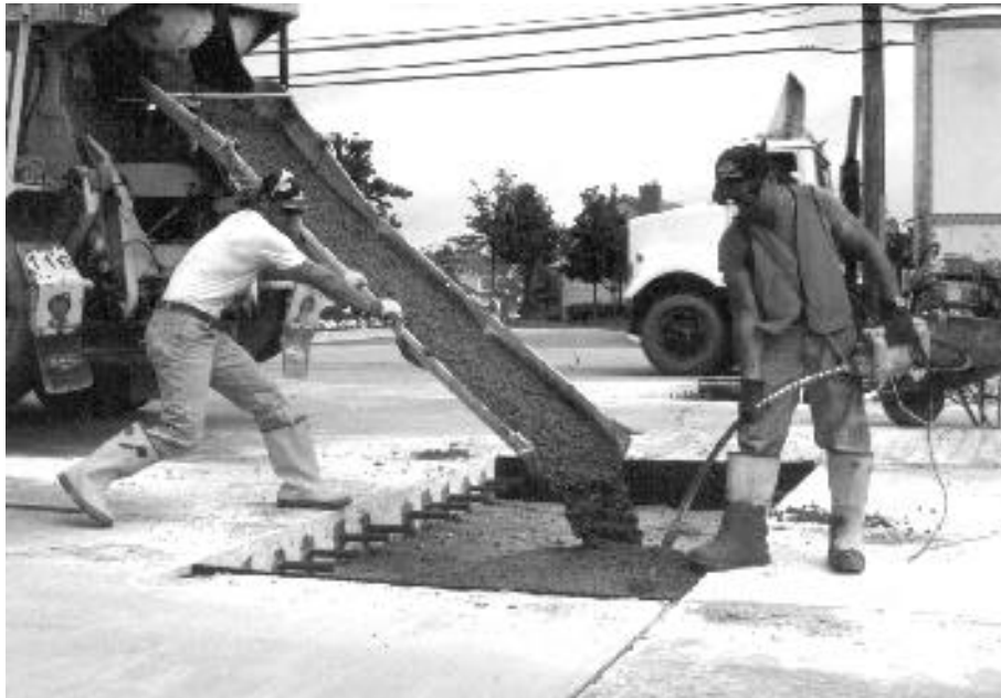
Figure 2: Placing concrete in full-depth repair [ACPA-TB020P]
